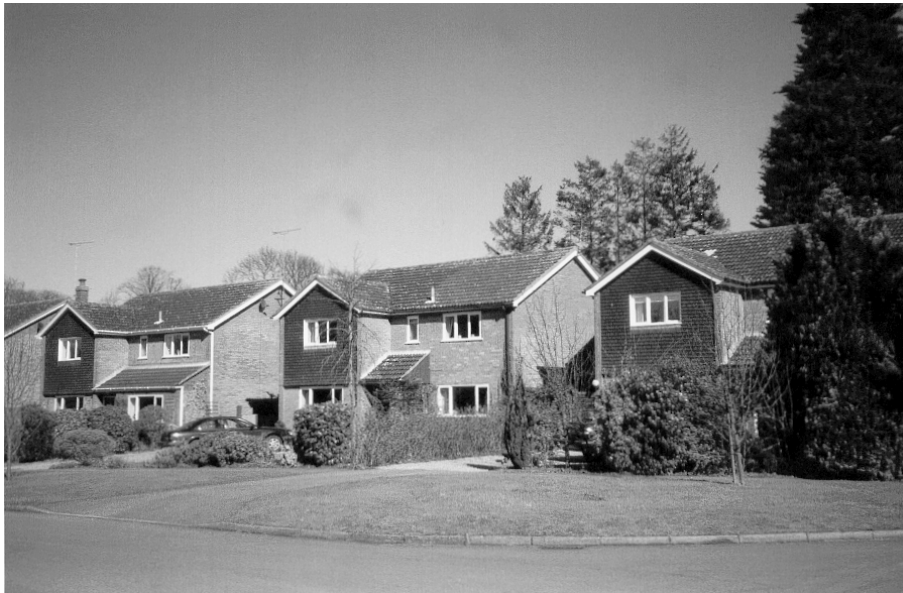
Where Birley's house stood is now the back gardens of these houses in Beech Way
